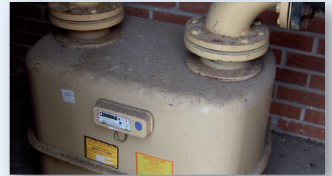
A standard gas meter
